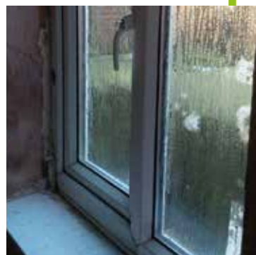
Condensation on windows
