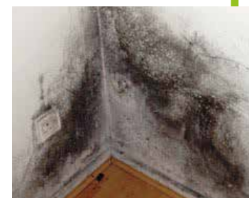
Mould on walls
