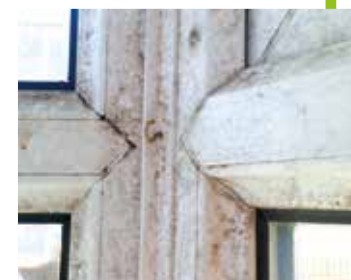
Mould on window frames
